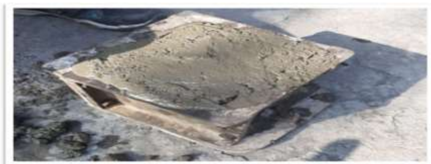
Fig 3.7 casting of cubes
